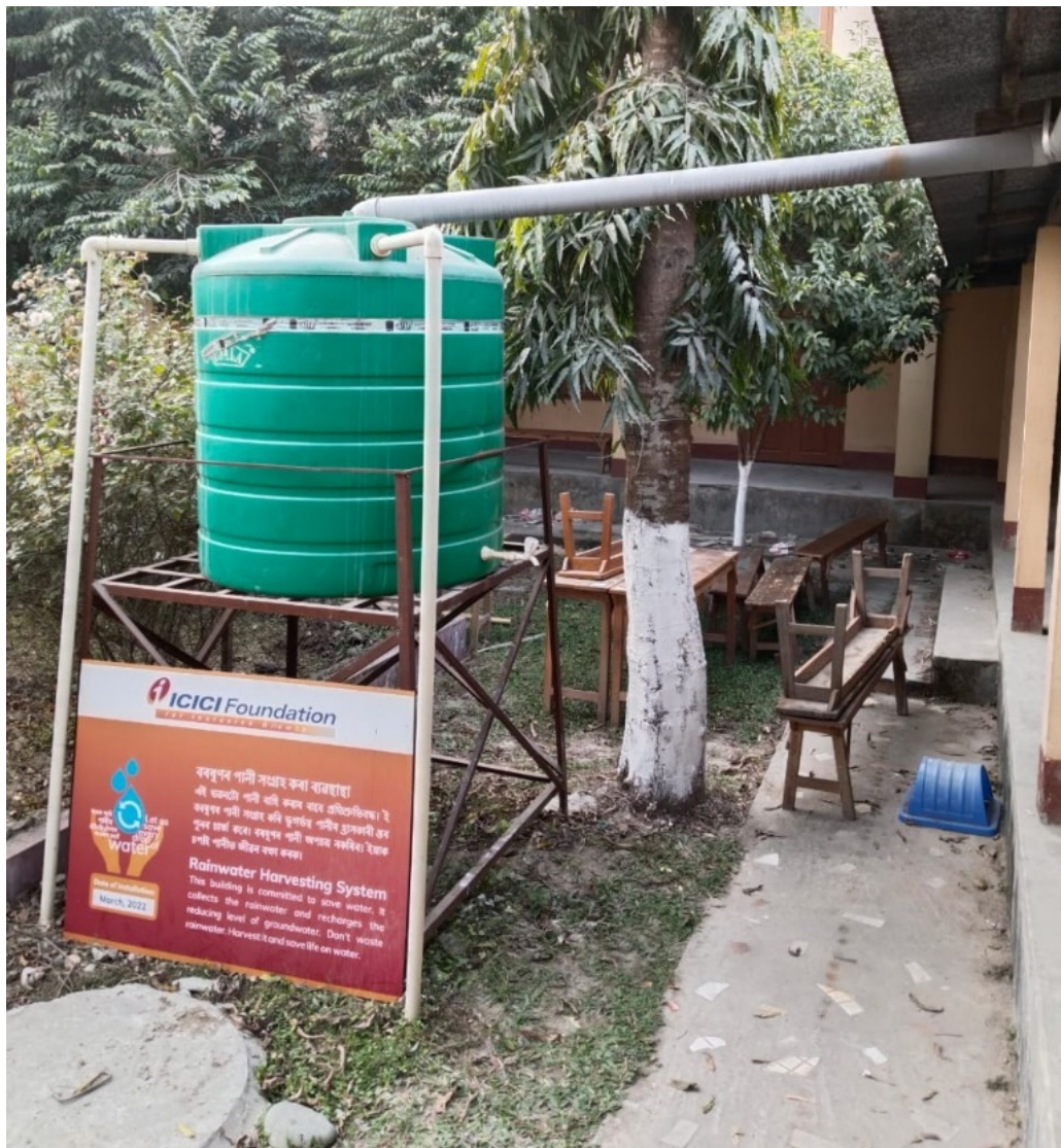
Rain water harvesting & ground water recharge set-II
